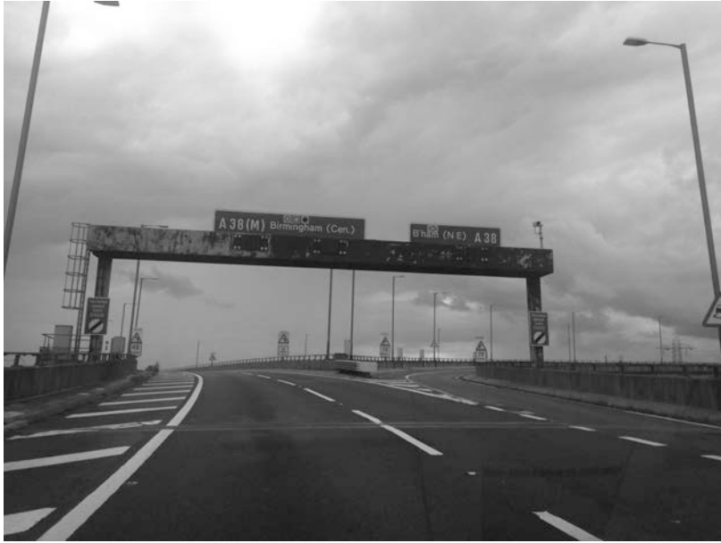
19. Intersection of A38(M) Aston Expressway and M6 motorway
